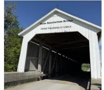
State Sanatorium Bridge
