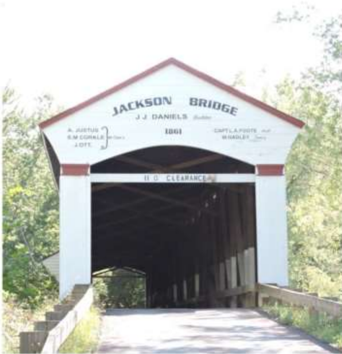
Jackson Covered Bridge over Sugar Creek, Parke County, IN Built 1861 by Joseph J. Daniels Double Burr Arch truss, 228 feet, 1 span
