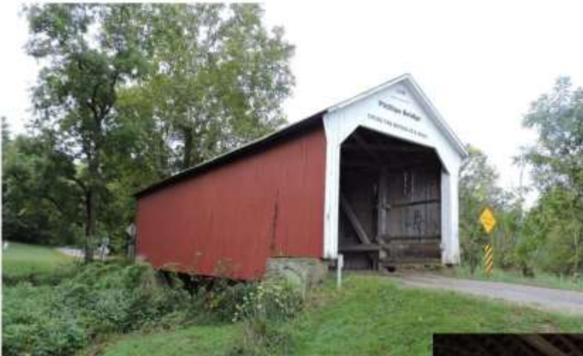
Phillips Covered Bridge over Big Pond Creek, Parke County, IN Built 1909 by Joseph A. Britton Multi Kingpost truss, 60 feet, 1 span
