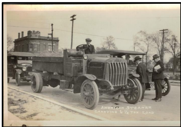
Carrying Six and Half ton load.
